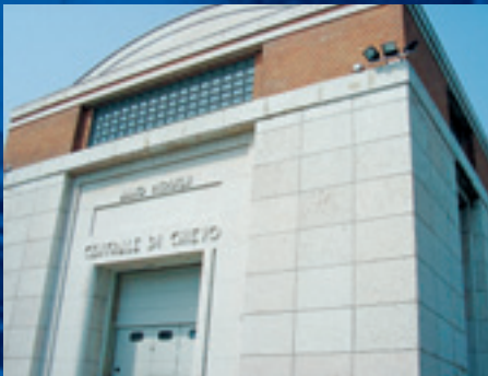
Detail of the historical building of the Chievo power plant.
