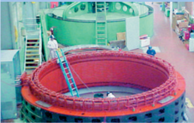
Completed stator rewind (Courtesy of Alcoa, Inc.)
