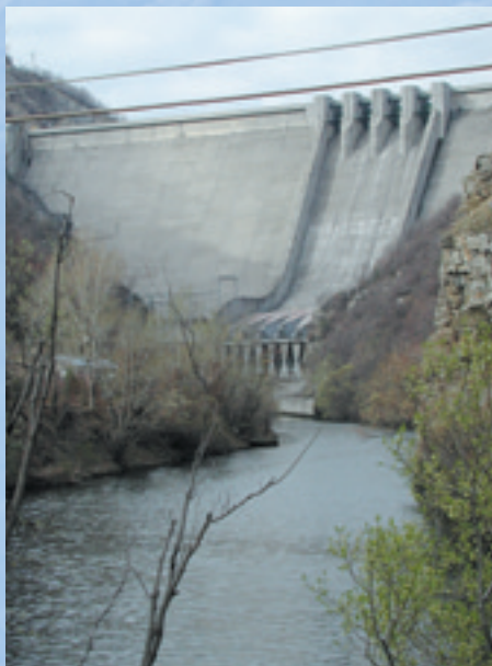
Dam with spillway at Orfeus reservoir
