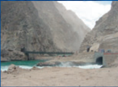
Laxiwa project site
