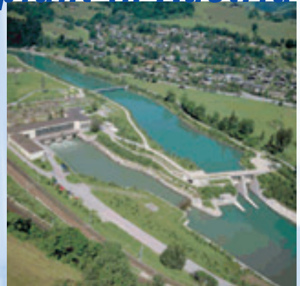
View of the hydro power plant
