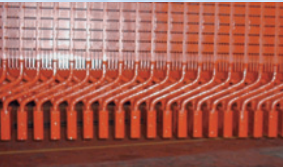
Before and after repair
