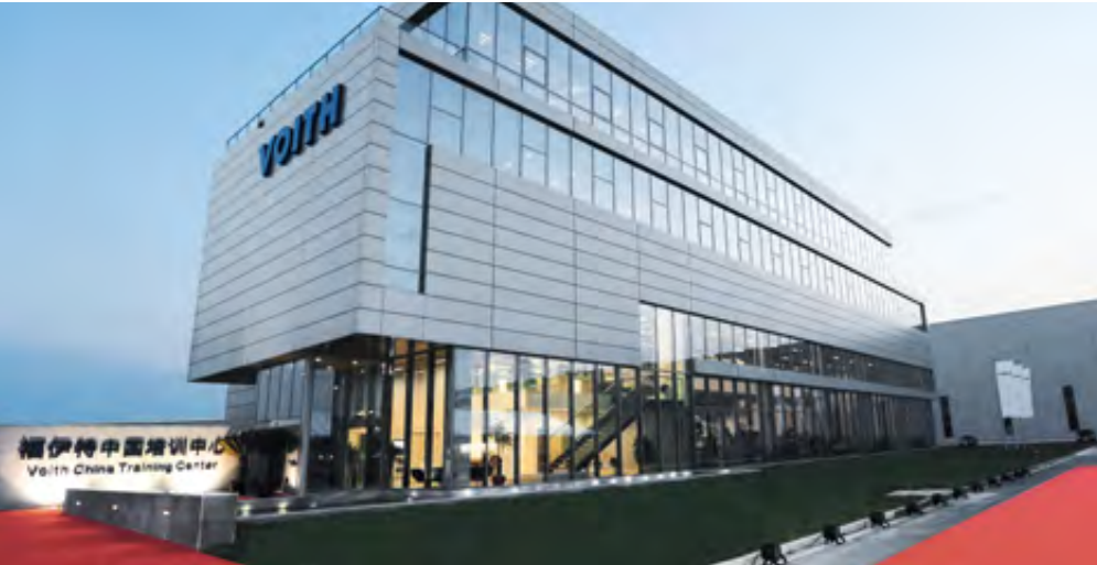
Das Voith China Training Center in Kunshan.
